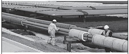
Polyguard's unique ReactiveGel® gel system reacts with elements in the steel to form an extremely thin, glasslike mineral layer on the steel surface. This mineral layer will not corrode.
