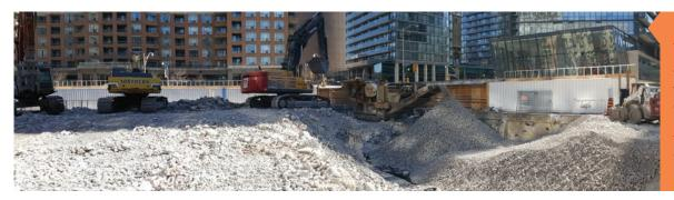
All the concrete recovered from the demolition was crushed onsite and used to backfill the basement cavity.
