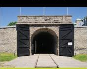
The Brockville Railway Tunnel, located beneath Brockville City Hall in downtown Brockville, ON, is the first railway tunnel built in Canada. The tunnel, which is 4.5 metres wide, 4.3 metres high and 525 metres long, was constructed from 1854 to 1860 in three sections, including a segment that required blasting through solid granite with gun powder. The last train passed through in 1969. Today, it's a local attraction.
