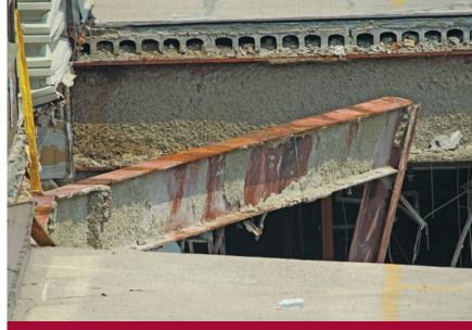
Norr Group found, in the course of its investigation, that severe rusting of a connection between a beam and column supporting the mall's rooftop parking lot was the main reason for the collapse.
