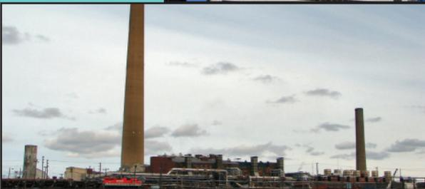
The Superstack in Sudbury, Ontario, is the tallest chimney in Canada at 1247 feet (380 metres) and is the second tallest freestanding structure, behind the CN Tower. Built in 60 days in 1970, it's located at Vale Inco's Copper Cliff processing facility and set to be dismantled in 2020.
