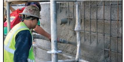
Installing concrete at a high velocity reduces costs and improves durability – that's the shotcrete advantage.
