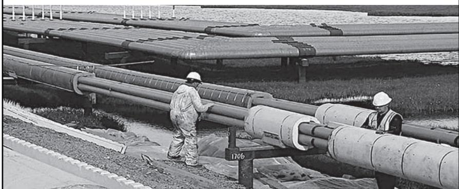
Polyguard's unique ReactiveGel® gel system reacts with elements in the steel to form an extremely thin, glasslike mineral layer on the steel surface. This mineral layer will not corrode.
