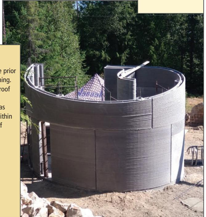
The assembled Fibonacci House prior to the roof framing. The structure's roof was made from wood, which was sourced from within 10 kilometres of the site.
