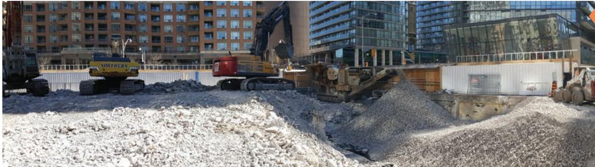
All the concrete recovered from the demolition was crushed onsite and used to backfill the basement cavity.
