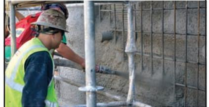
Installing concrete at a high velocity reduces costs and improves durability – that's the shotcrete advantage.
