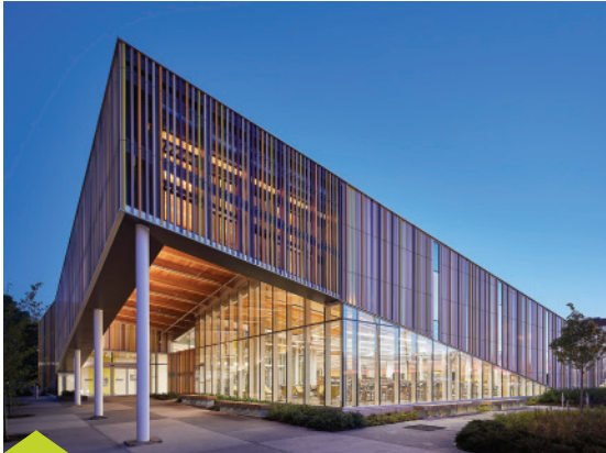
Albion District Library in Etobicoke, Ontario, designed by structural engineering firm Blackwell, is an Ontario Wood WORKS! Wood Design Awards winner.
