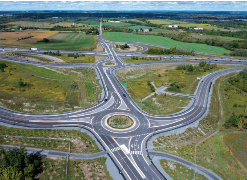
An example of the Ministry of Transportation of Ontario's integration of roundabouts on Ontario's highways, used to help calm traffic. This roundabout is at Holt Road and Highway 401 in Clarington, Ontario. Photo: MTO
