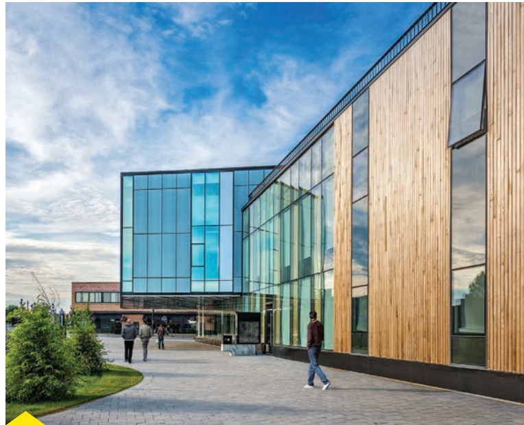
AECOM won the Wood WORKS! Institutional Wood Design Award over $10 million for work on the McEwen School of Architecture in Sudbury, ON. Photo: Bob Gundu
