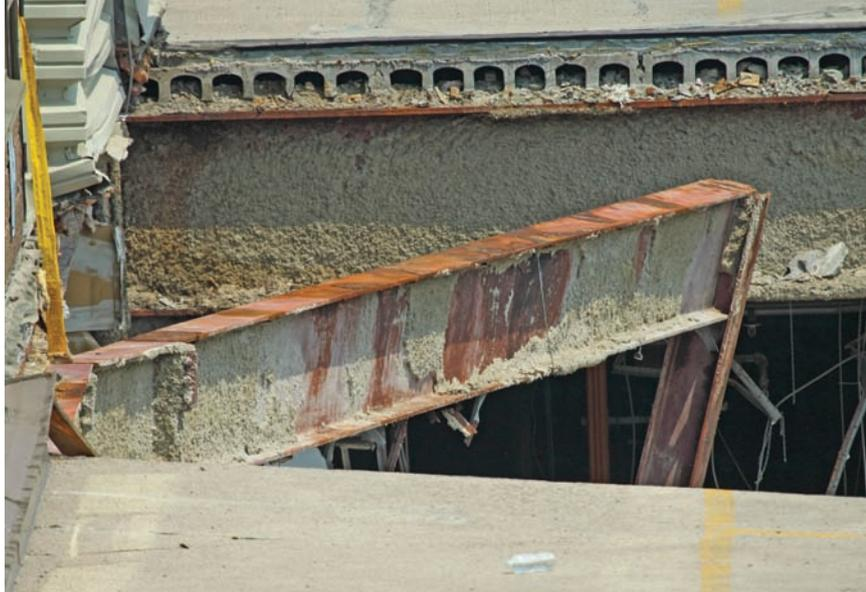
Norr Group found, in the course of its investigation, that severe rusting of a connection between a beam and column supporting the mall's rooftop parking lot was the main reason for the collapse.
