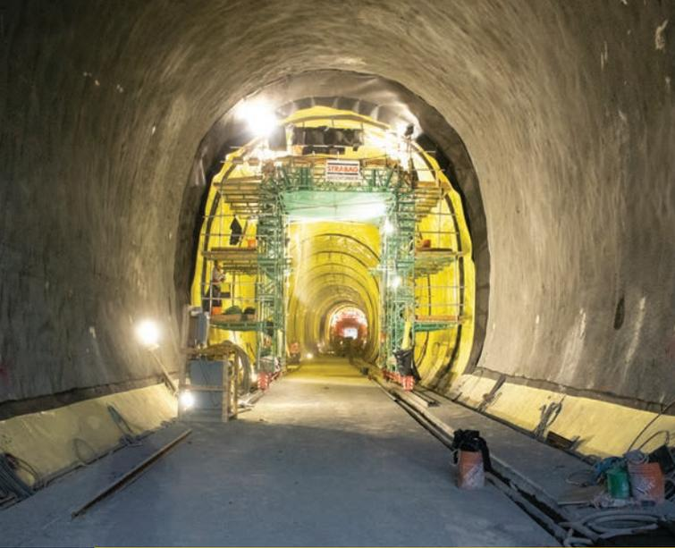
The 401/409 twin rail tunnels are fully waterproofed. The waterproofing system consists of a PVC waterproofing membrane installed between the initial lining and cast-in-place final lining. Photo: Metrolinx
