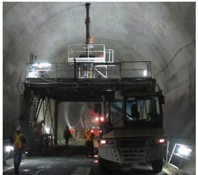
Concrete was dropped over 100 metres from the surface down to the Niagara Tunnel, where it was remixed and loaded into concrete trucks, which delivered it to the final lining operation.
