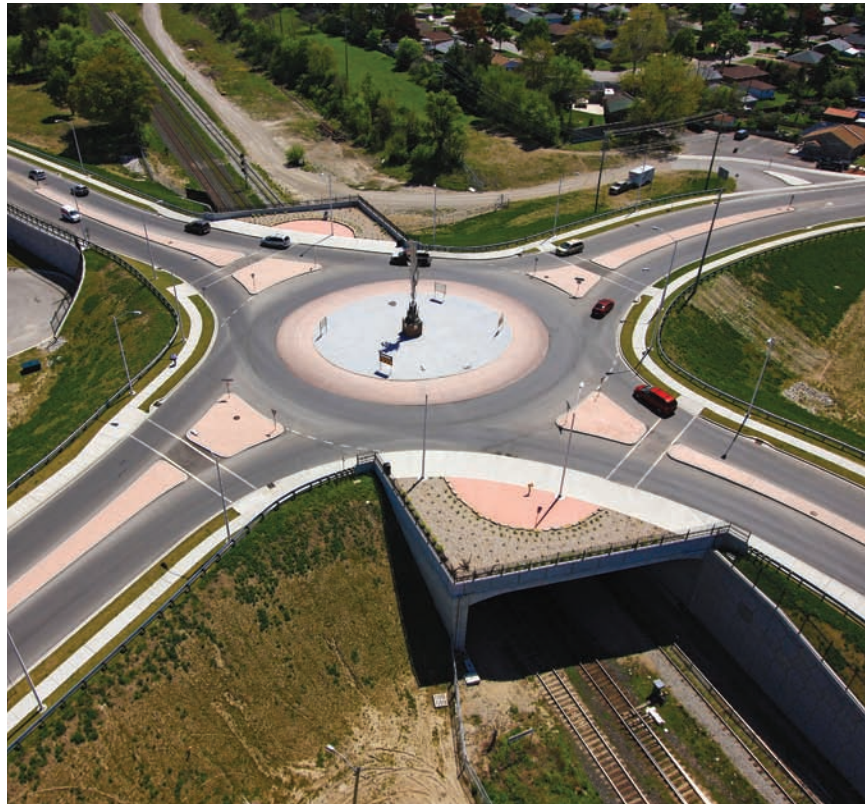
London’s Charley Fox Memorial Overpass—the first of its kind in Canada—is an 86-metre-long elevated roundabout built over CN rail tracks.
