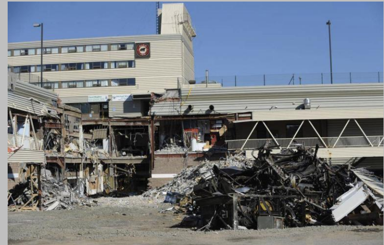
Algo Mall Collapse in Elliot Lake
