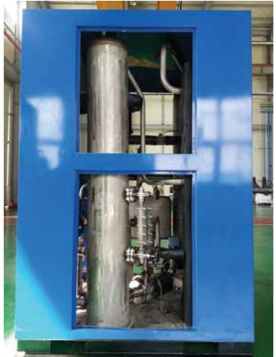
A side view of one of Thermalfrost’s chillers, which uses heat to generate cooling. It’s currently being used for industrial and commercial purposes like fishing vessels and refrigerated trucks and could one day replace mechanical vapour compression refrigeration, which consumes electricity and uses pollution-causing refrigerants.
