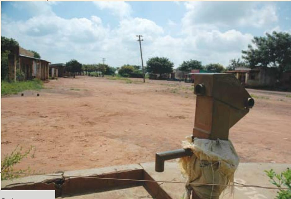
Broken hand pump: Something as simple as a broken bearing can eliminate water for thousands in rural Malawi.
