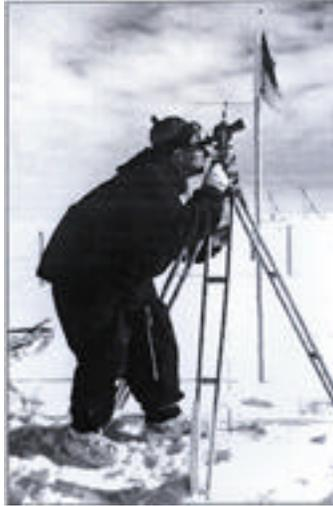
◀ Joe MacDowall, P.Eng., leader of the Royal Society International Geophysical Year Antarctic Expedition, is shown here using a theodolite (a survey telescope) on the Brunt Ice Shelf by the coast of the Weddell Sea in 1957. Theodolite observations of the sun and stars were used to track the seaward movement of the ice shelf.
