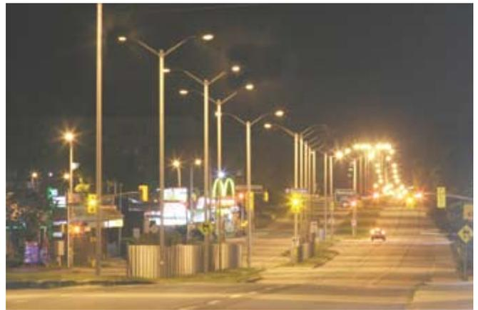
Figure 2: Re-lamping during infrastructure renewal is a cost-effective way to upgrade street lighting. The improved visibility without glare (foreground) is evident compared to the unshielded fixtures in the distance. However, the glare from commercial lighting continues to affect visibility and the visual clutter decreases safety by distracting drivers even after businesses have closed.
