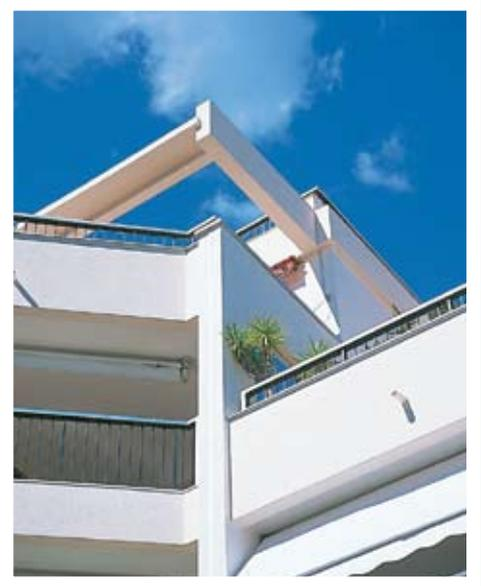
Lotusan exterior coating, developed by Sto Corp., possesses a highly water-repellent surface similar to that of a lotus leaf, where water droplets roll off and take dirt with them (top). The photo above shows a building with Lotusan coating, where water and dirt flow off immediately and the facade remains dry and attractive.
