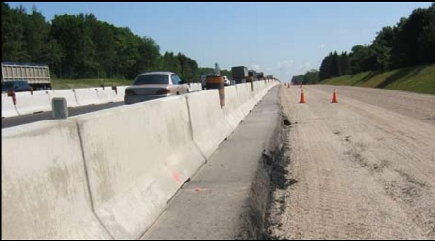
Twenty-four lane-kilometres of Highway 401 were reconstructed with perpetual pavement, a heavy-duty pavement alternative designed to withstand heavier loads and resist structural failure for at least 50 years.
