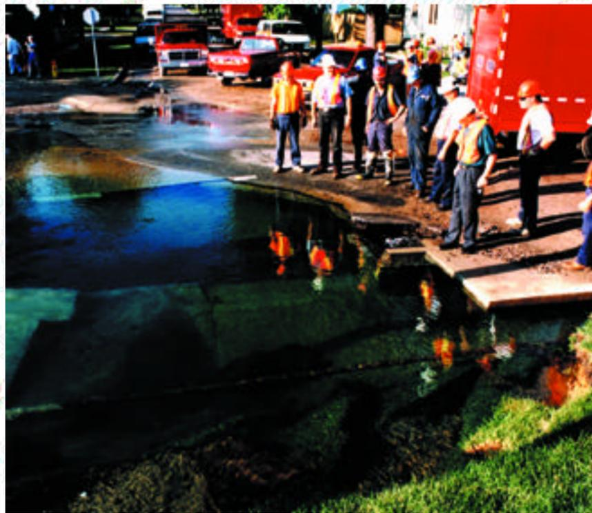
This recent watermain break in Sarnia turned into a flood after the line ran for eight hours because staff were unable to locate a valve buried under asphalt. As a result, a length of road base was damaged, spoiling previous work. Such problems can be prevented by computer systems that keep inventories of infrastructure and enable good record keeping. Photo: Glenn Ogilvie, courtesy of The Observer.
